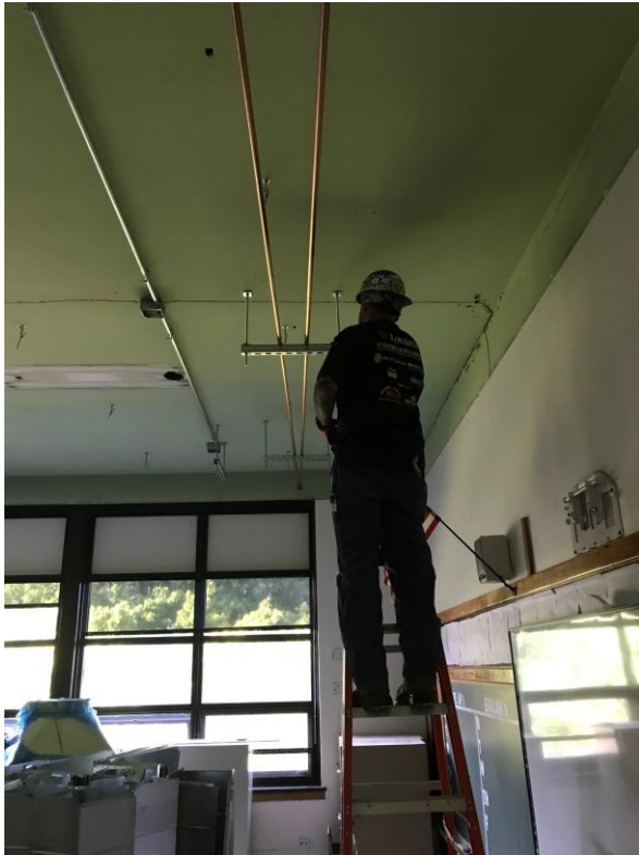
Hot water pipe installation
