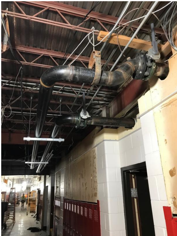
Hot water pipe installation
