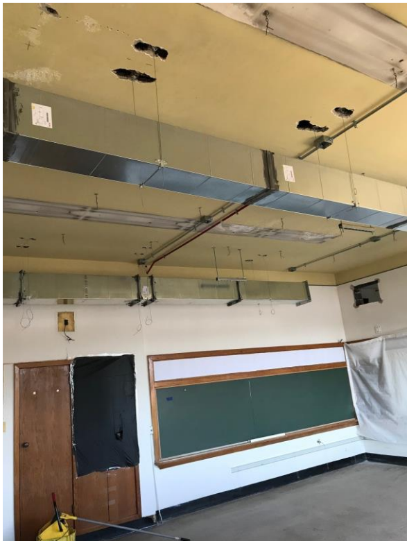
2 nd floor duct installation
