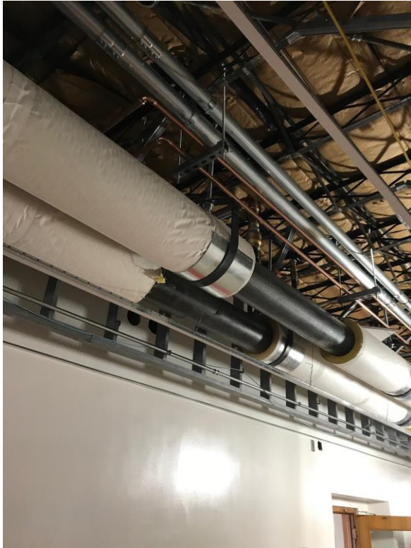
2 nd floor water main installation
